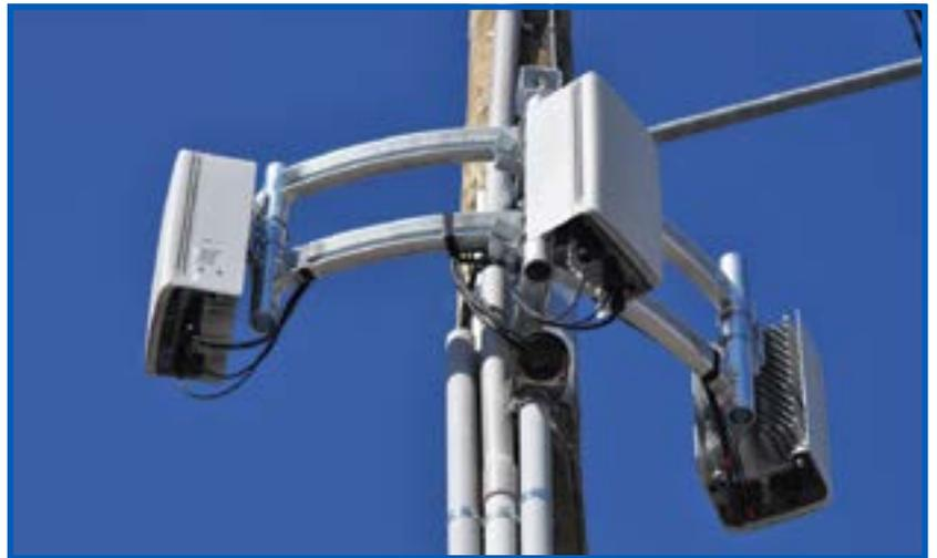
97-5GWDMTHGN1-A installation with (3) customer-supplied 5G radios
